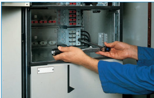
Safe connection of outgoing cables is possible under live busbar conditions.
