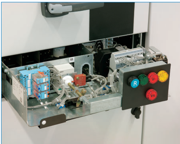
Capitole 40 cubicle showing partly withdrawn motor starter tray.
